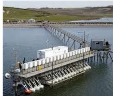
Figure 19: WaveStar installed at Nissum test site.
