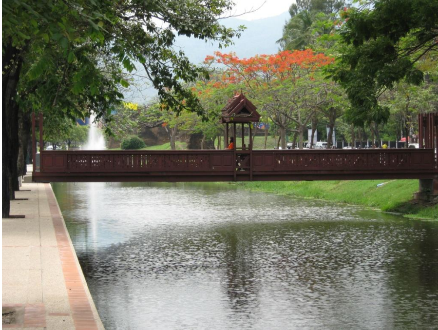
Bridge in Chiang Mai
