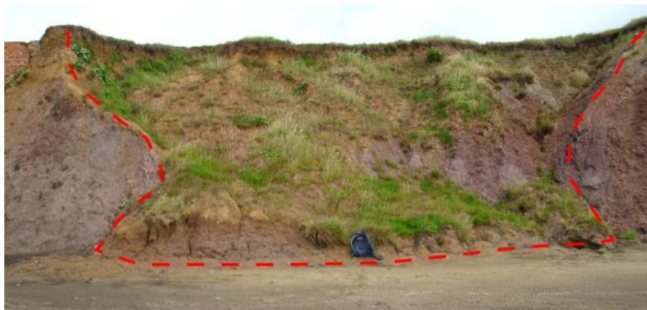
Figure 3.6 Shallow Translational (planar) landslide in Sandown Bay, failure occurring near top of cliff (2). 40L back pack for scale.
