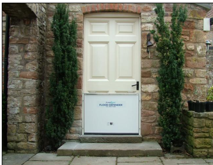
Figure 13: A typical PLP measure (door barrier) used to prevent water ingress through a door frame (UK Flood Barriers Ltd, 2015)
