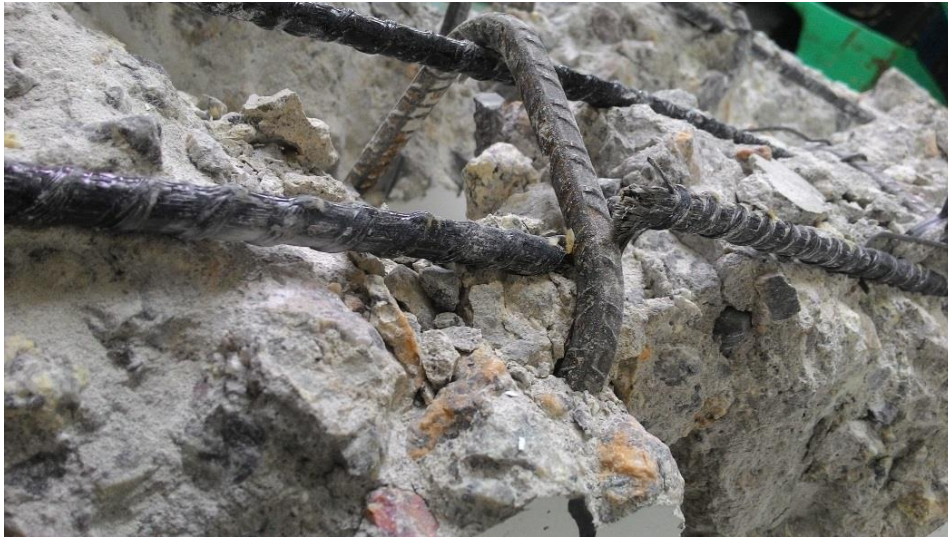
Photo 12: Beam B3 Reinforcement Failure.
