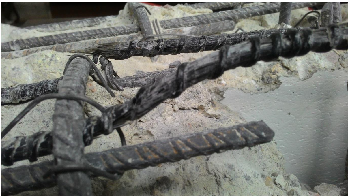
Photo 11: BFRP Rebar Reinforced Concrete Beam B2: Reinforcement Failure.
