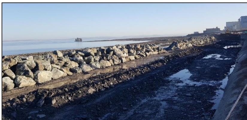
Figure 1: Rock armour placed at Hinkley Point C prior to construction
